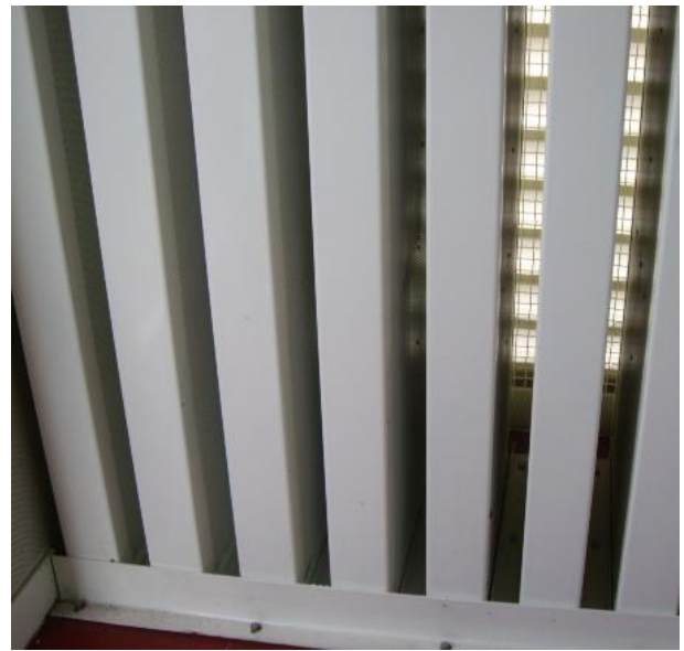
Inlet attenuator detail 85dBA @ 1M
