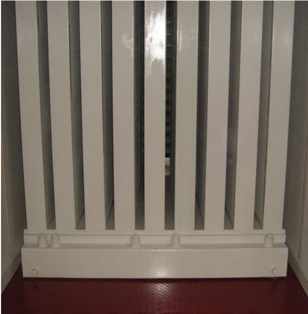
Inlet attenuators mounted on day fuel tank
