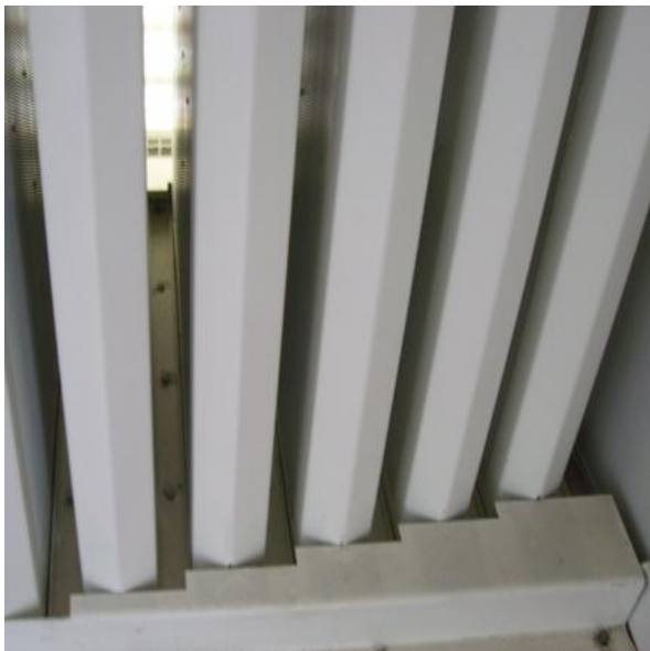
Outlet attenuator detail 85dBA @ 1M
