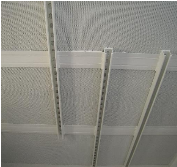
Multi position unistrut for easy exhaust and light fitting
